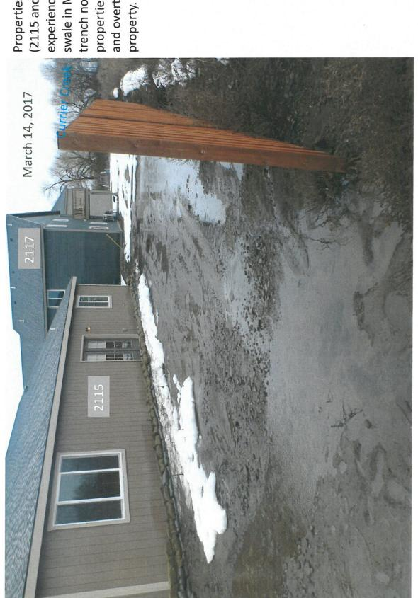
Properties on Creeksedge Way (2115 and 2117) that experienced flooding from the swale in March 2017. The trench north of their properties was at full capacity and overtopping into their property.
