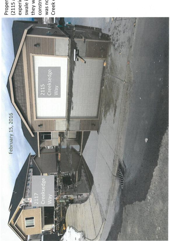
Properties on Creeksedge Way (2115 and 2117) also experienced flooding from the swale in February 2016 while they were still under construction. This flood water was not the result of Currier Creek overtopping its banks.
