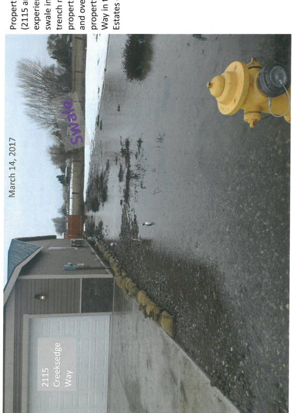
Properties on Creeksedge Way (2115 and 2117) that experienced flooding from the swale in March 2017. The trench north of their properties was at full capacity and overtopping into their property toward Creeksedge Way in the Currier Creek Estates development.
